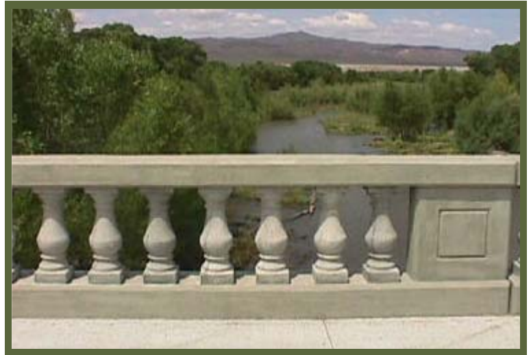
The Winkelman Pedestrian Bridge
